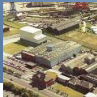
Heraeus Conamic UK Ltd., Wallsend facility, UK
